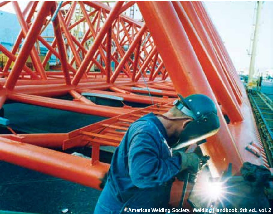
Shielded metal arc welding (or “stick welding”)
