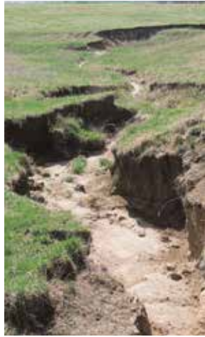
GULLY EROSION FROM UNCONTROLLED RUNOFF
