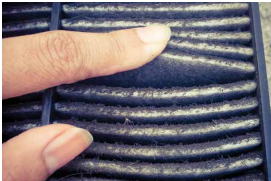
Checking the air filter
